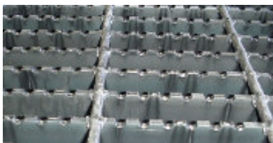
Serrated Steel or Aluminum Grating on 24 ft. of slope
